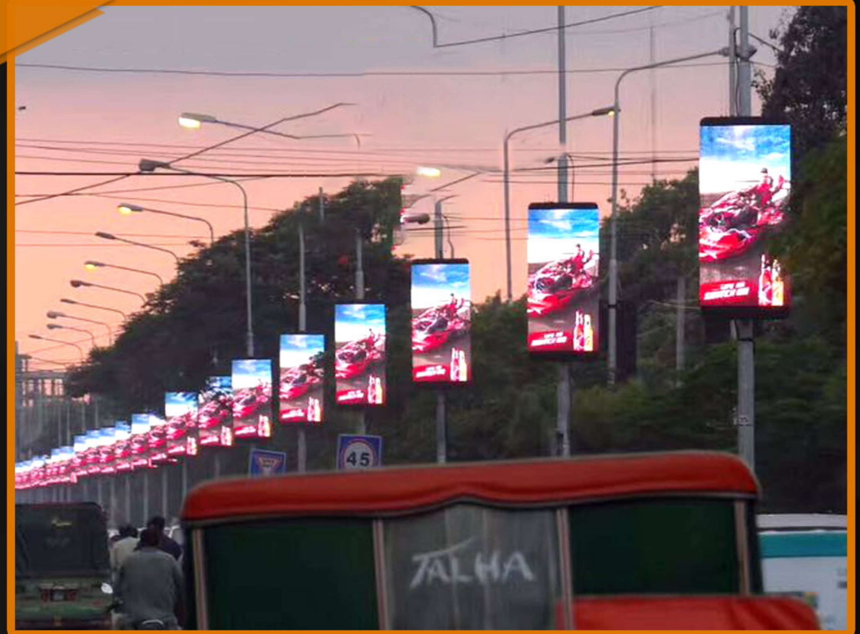
Lamp-Pole Display in Jiangsu 224 m 2
